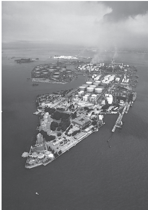
Part of a petrochemical plant in Singapore
